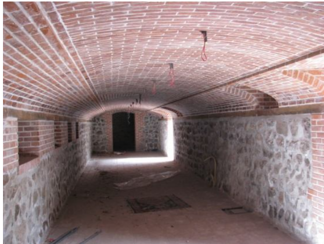
Figure -1 use of the basement in house of Sadeghi
